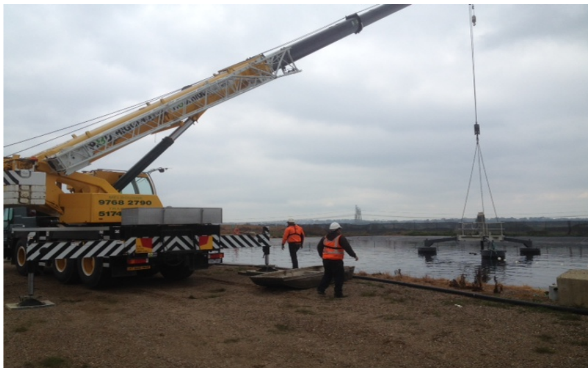
LIFTING AERATOR INTO LAGOON FROM SERVICE PAD
