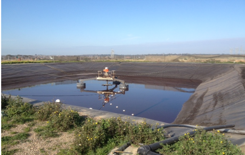
AERATOR IN LAGOON AT END OF DISCHARGE, RESTING ON PAD, STARTING TO FILL.
