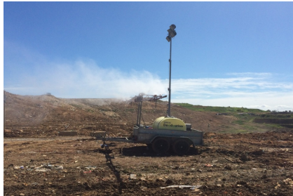
'Batwing' Odour Neutralising System at the active cell
