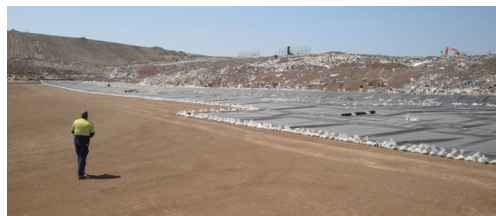
Internal waste batter – Lining example
