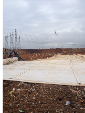
ADC – Landfill Tarp Cover with Odour suppression system
